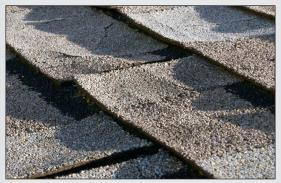
**Curling/Cupping** – This is the result of normal weathering of the asphalt shingle.
