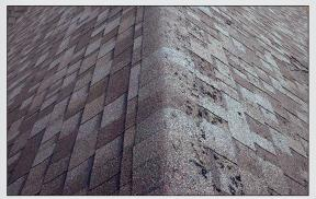
**Hail** – The number, size and hardness of the hailstones can vary tremendously within a small locality. Velocity and direction of the wind are also factors.
