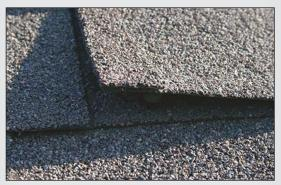
Nail Pop – An elevated nail that can push a portion of the shingle off the roof plane. Over time, this pop can cause a hole in the shingle.
