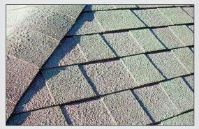
Blisters – Small bubbles or crater-like holes generally. Blistering can result from the manufacturing process or from roof ventilation issues and are not caused by hail. Blisters can eventually cause granule displacement.
