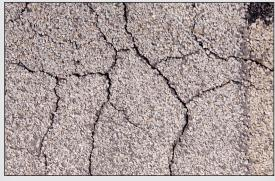
**Cracking** – Web-like pattern of cracks in surface of shingles due to natural weathering.
