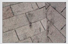
**Footfall** – Potential loss of granules caused by walking on a roof.
