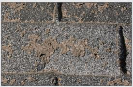
Flaking – As the natural weathering of shingles continues, small chunks of the granule coating begin to delaminate from the mat.
